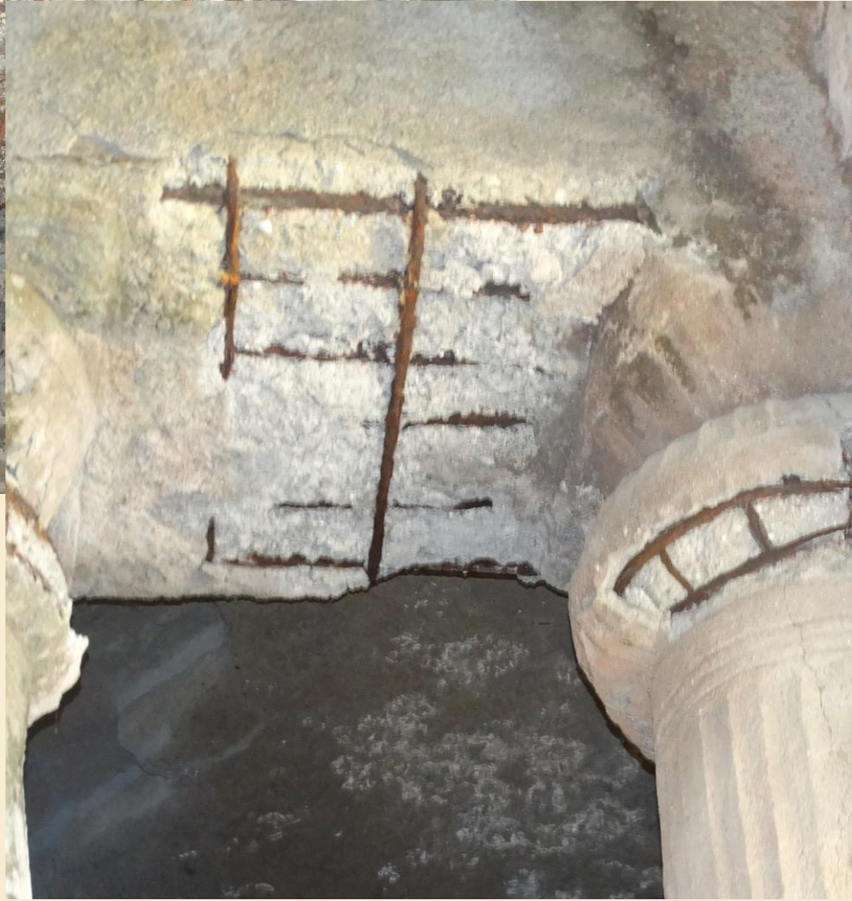
Some example of reinforcement of the pillars made with concrete and iron bar, net, spiral, on 1970. The Temple is on a island, by the sea. The corrosion cannot be refrained by the limited concrete cover. 1962
