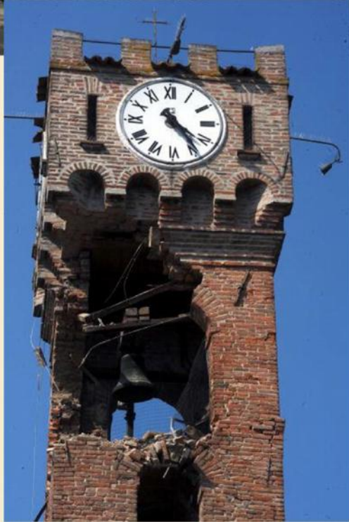
Pictures from the damage caused by the L'Aquila earthquake, 2009, Italy
